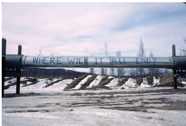
Figure 2: Graffiti on the recently-completed pipeline north of Fairbanks, 1977-1978. Source: Richard Seifert.
