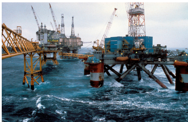
Figure 2: Alexander L. Kielland (right) before the disaster. The rig was contracted by Stavanger-based company A. Gowart-Olsen & Co in 1973. It was a semi-submersible Pentagon drilling rig with five legs, specifically designed for demanding weather conditions. The rig was built at the CFEM shipyard in France and completed in June 1976. Due to a lack of drilling assignments, it was converted into an accommodation rig and was solely used for lodging throughout its lifespan. Photo: ConocoPhillips / Norwegian Petroleum Museum (NOMF-02663.652)
